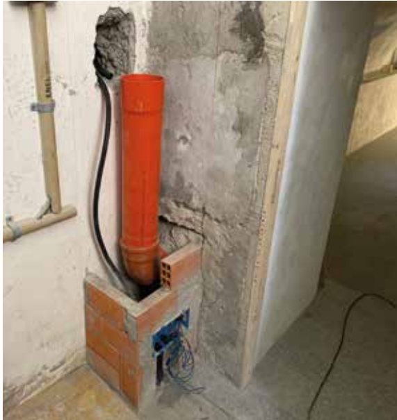
Preparation of extraction point
