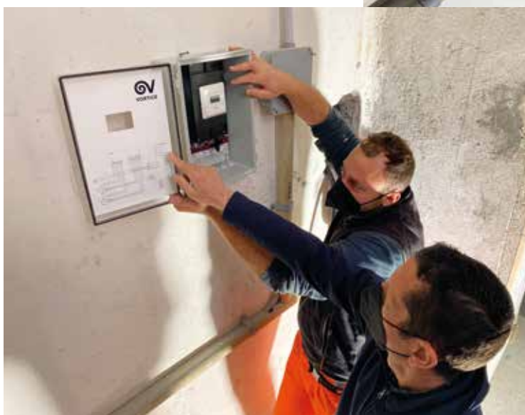
SICURBOX control unit installation for control, monitoring and management.
